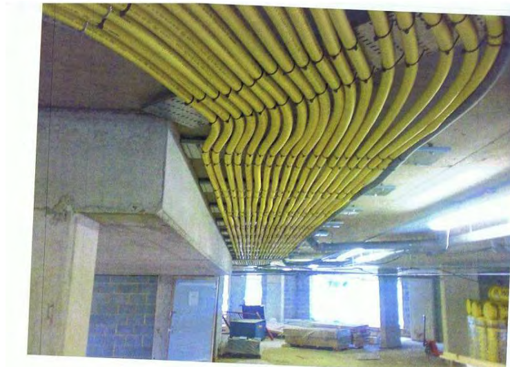
Long Length of CSST Used in UK Provided by Omegaflex
