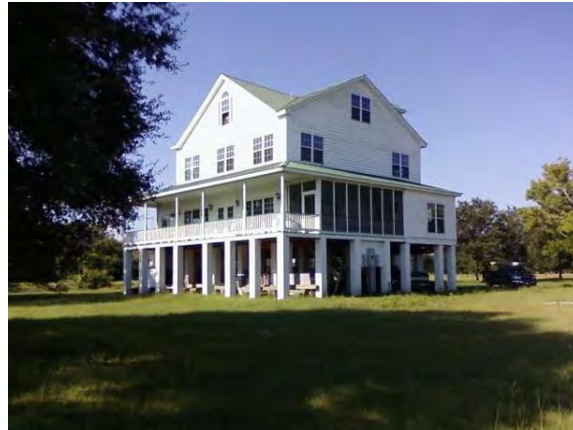
General View of the House Showing the Lack of Lightning Electromagnetic Shielding Provided by the Structure
