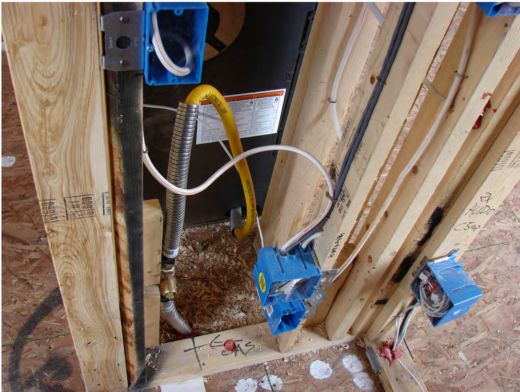
CSST is run Outside a Metal Tube for a Short Distance
