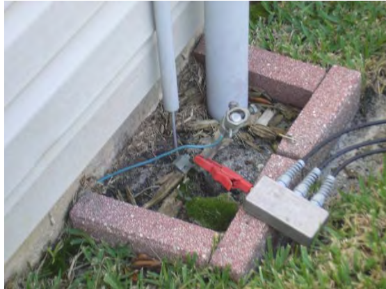
Grounding Electrode Test Point Configuration
