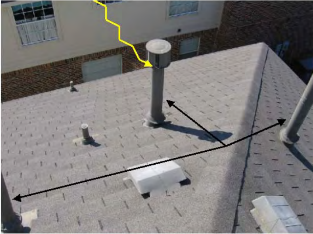
View of the Metal Flue Pipes on a Roof
